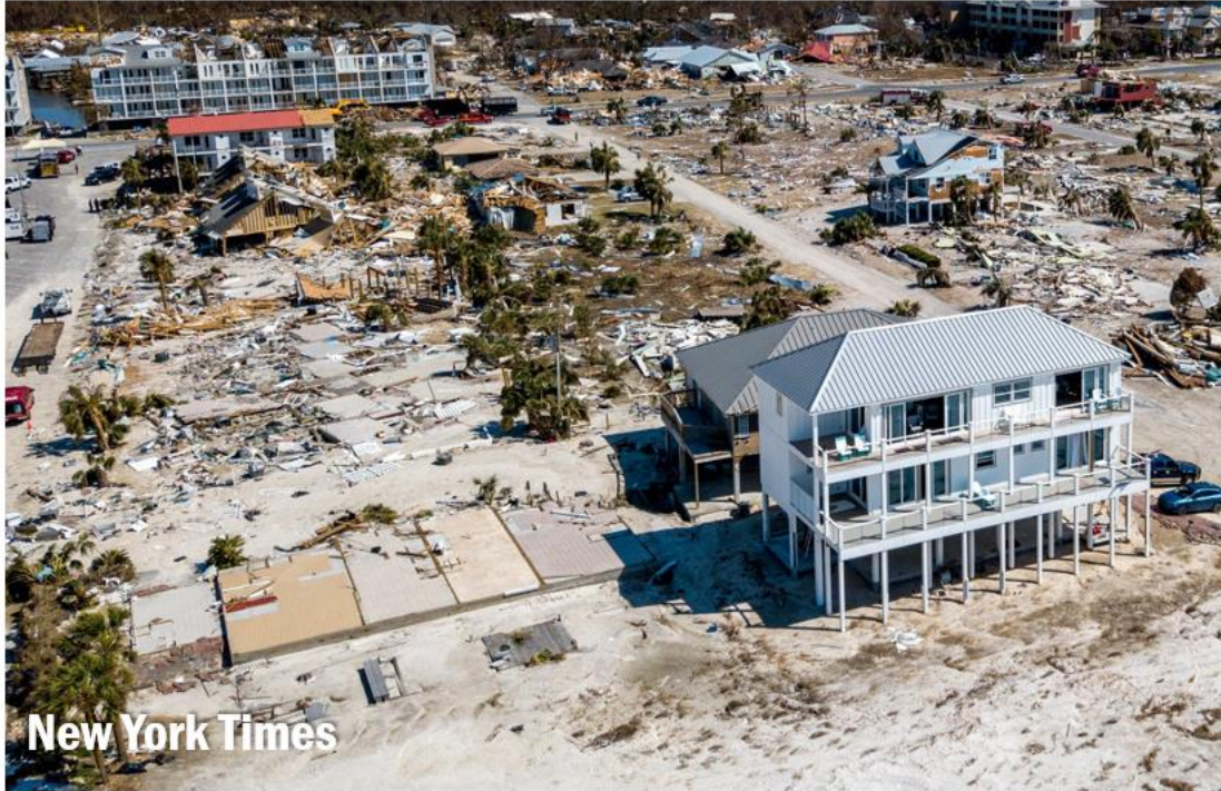
Mexico Beach after Hurricane Michael
