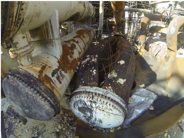
Figure 3 Reboiler, post-accident
