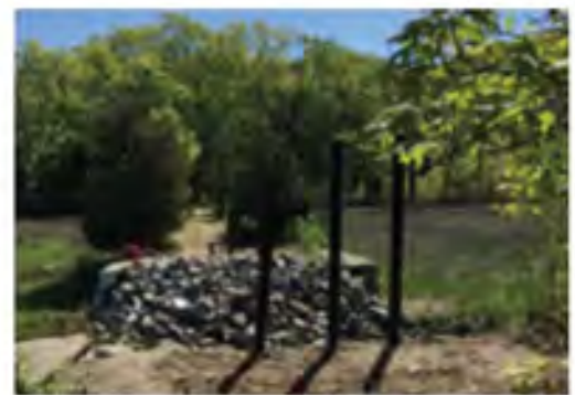
6 helical anchors installed
