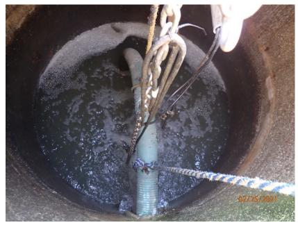
Description: Lift Station #8 was not operational. The manhole across North 75<sup>th</sup> Street had a pipe across it from which a submersible pump was hanging. The manhole contained water.
