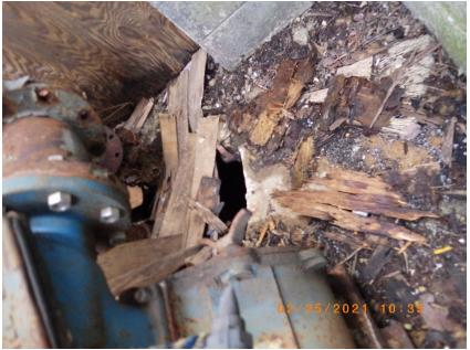
54: CFCD0007\_20210225 Description: Lift Station #13. Lift station wet well cover damaged and open to the elements. Location: Lauralee Dr., dirt access road between homes and field to the east. Camera Direction: East Date/Time: 02/25/21/10:35 A.M.
