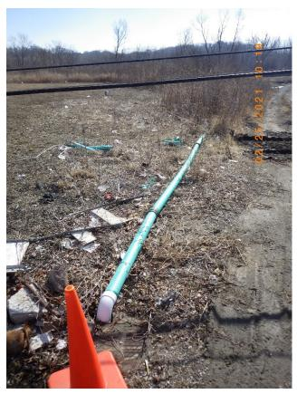
34: CFCD0005\_20210225 Description: Lift Station #20. Bypass pipe from lift station entering manhole on Missouri Ave. Location: Missouri Ave, dirt access road just north of Rt. 13. Camera Direction: Southeast Date/Time: 02/25/21/10:19 A.M.
