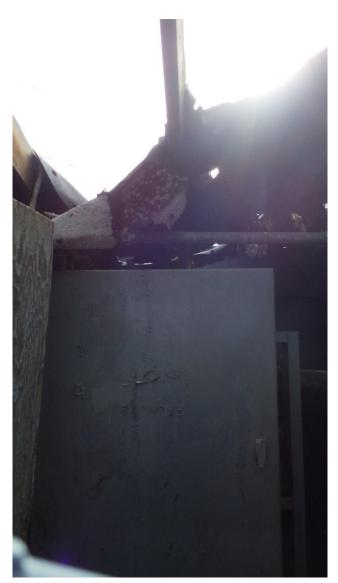
55: CFCD0008\_20210225 Description: Lift Station #13. Ceiling of lift station building damaged and open to the elements. Location: Lauralee Dr., dirt access road between homes and field to the east. Camera Direction: South Date/Time: 02/25/21/10:35 A.M.
