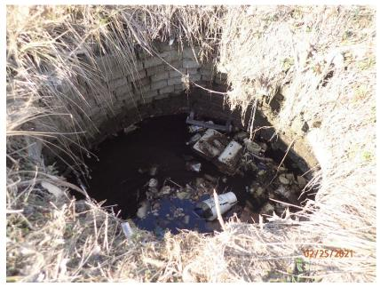
Description: Just southwest of Lift Station #7 is an uncovered brick manhole that was filled with water. EPA told the Manager of Commonfields of Cahokia about this safety hazard on 2/25/21. Location: South side of North 73<sup>rd</sup> Street between Dorris Street and State Street. Camera Direction: Down Date/Time: 02/25/21/9:32 A.M.
