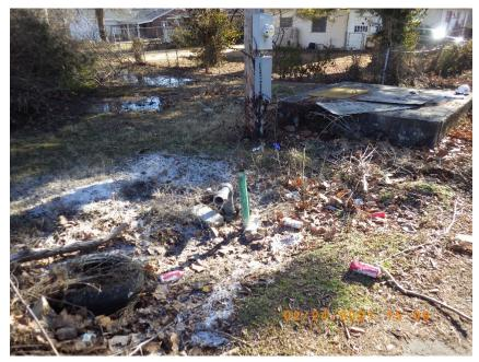
289: CFCD0002\_20210224 Description: Toilet paper debris surrounding a discharge pipe, fitted for a hose connection, for Lift Station #21. Location: Lift Station #21, Ash St between Lake Dr. and Park Place. Camera Direction: Southeast Date/Time: 02/24/21/3:09 P.M.
