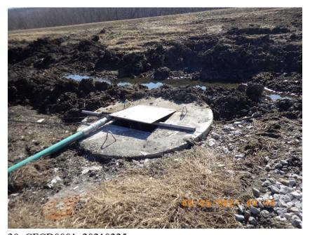
30: CFCD0001\_20210225 Description: Lift Station #20. EPA noted that the vault cover was open to accommodate a pipe used to support a bypass pump. Note bypass piping. Location: Missouri Ave, end of dirt access road just north of Rt. 13. Camera Direction: Southeast Date/Time: 02/25/21/9:48 A.M.
