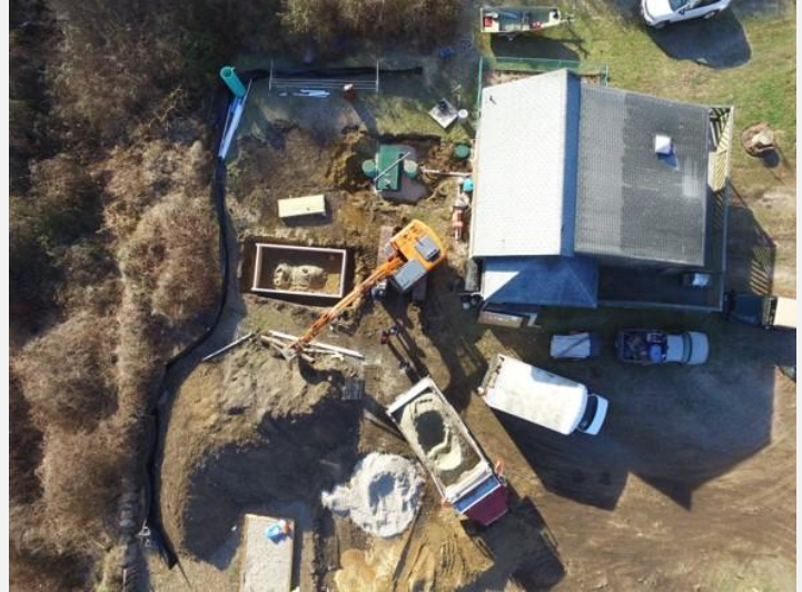
A nitrogen-reducing onsite wastewater treatment system is installed to replace a traditional septic system less than 100 yards from a coastal wetland
