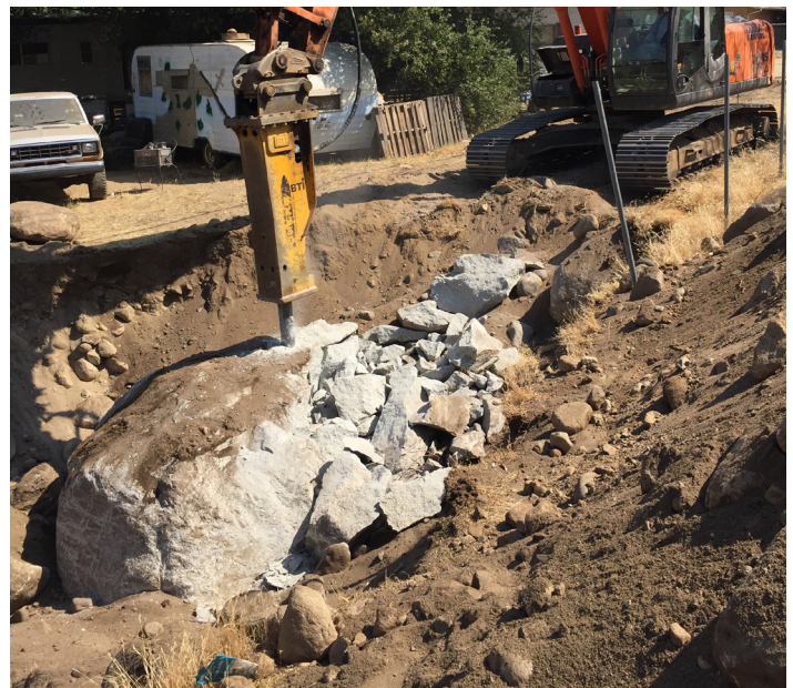
Tule River Rock Excavation
