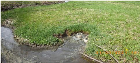
1: RIMG0051 (Photo cropped to remove Personal Identifiable Information) Description: Cleanout was discharging sanitary waste during dry weather. Location: East of North 80<sup>th</sup> Street. Camera Direction: Northwest Date/Time: March 31, 2021 / 11:21 A.M.
