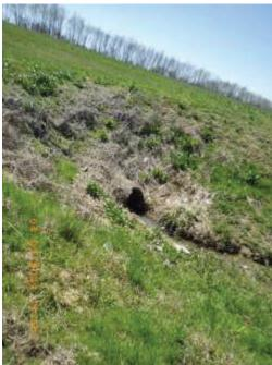
Description: outfall pipe inlet under the berm. Conveys stormwater from a ditch north of the berm to Harding Ditch.
