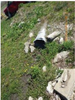
Description: inlet of metal pipe heading under the berm and to the outfall on Harding Ditch. Location: Station #8. MESD parcel along Harding Ditch, 90.1128622°W; 38.5533183°N Camera Direction: 85°
