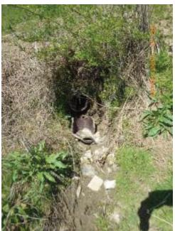
5: MESD0005 Description: outfall appeared to be damaged and was not flowing. Location: Station #2. MESD parcel along Harding Ditch, 90.1329908°W; 38.5461629°N Camera Direction: 328° Date/Time: April 1, 2021; 12:30 CT
