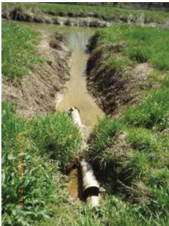
Description: outfall pipe was seperated from the pipe heading under the berm. Location: Station #6. MESD parcel along Harding Ditch, 90.1167107°W; 38.5506571°N Camera Direction: 162° Date/Time: April 1, 2021; 13:18 CT
