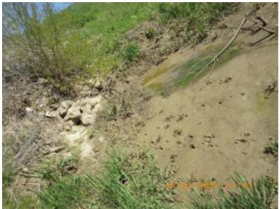
Description: outfall to Harding Ditch. The outfall appeared to be partially blocked by rocks and debris.
