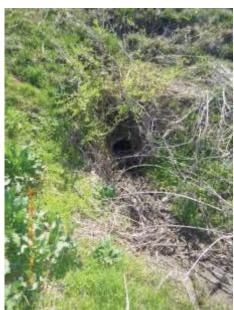
Description: outfall pipe inlet under the berm. Conveys stormwater from a ditch and field north of the berm to Harding Ditch.
