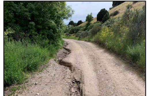
Example of erosion along City Creek Rd.
