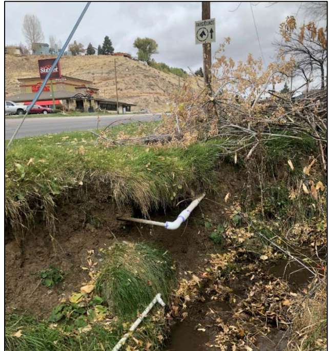
Severely eroded bank of Pocatello Creek.
