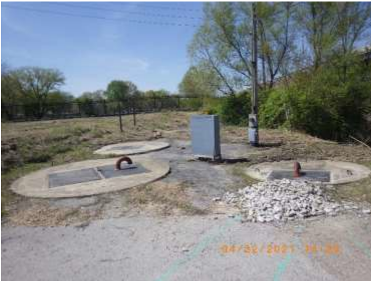
27: VCAH20017 Description: Lift Station #6, known as Cooper Station. Note cobbles filling in ground collapse in front of inflow vault. Location: Cooper & IL Rt 157 Camera Direction: 326° Date/Time: 4/22/21; 2:29 p.m.
