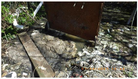
Description: Lift Station #5 – Lifted wet well cover. Wet well was full and the edge of wet well
