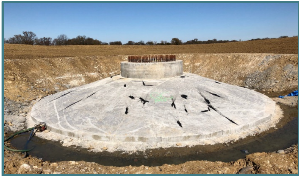
Completed base of wind turbine
