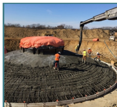
Pouring base of wind turbine
