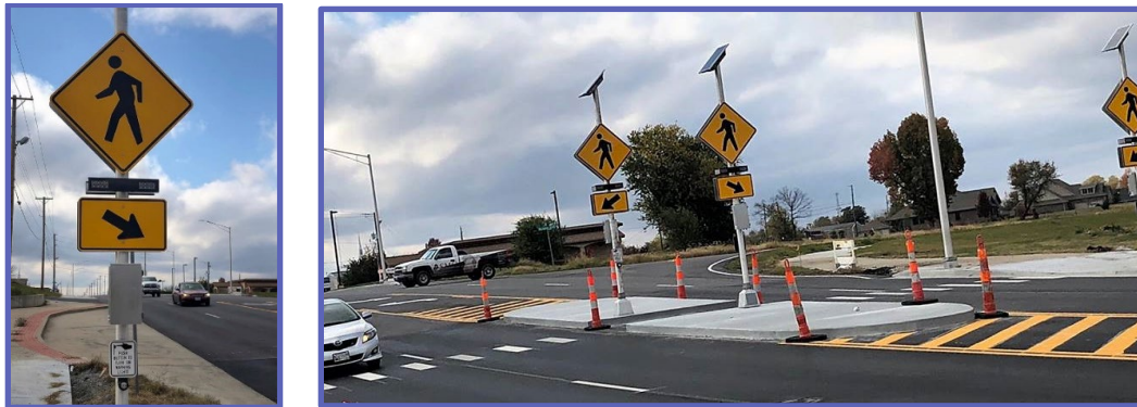
New RRFB pedestrian crossing installed on 20 th Street, Joplin, MO
