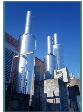
CWEP new exhaust stacks housing catalytic converters
