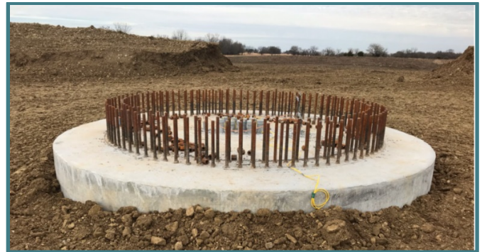
Graded base where wind turbine will attach
