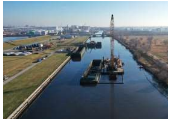
Lake George East Project dredging. (Credit: Kokosing Industrial, Durocher Marine Division).
