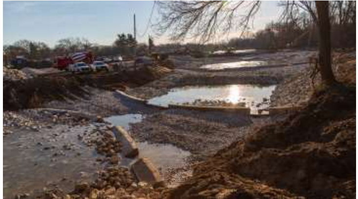
Construction of the Deep River rock riffle project
