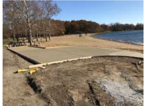
Construction of ramp to an ADA-compliant launch.
