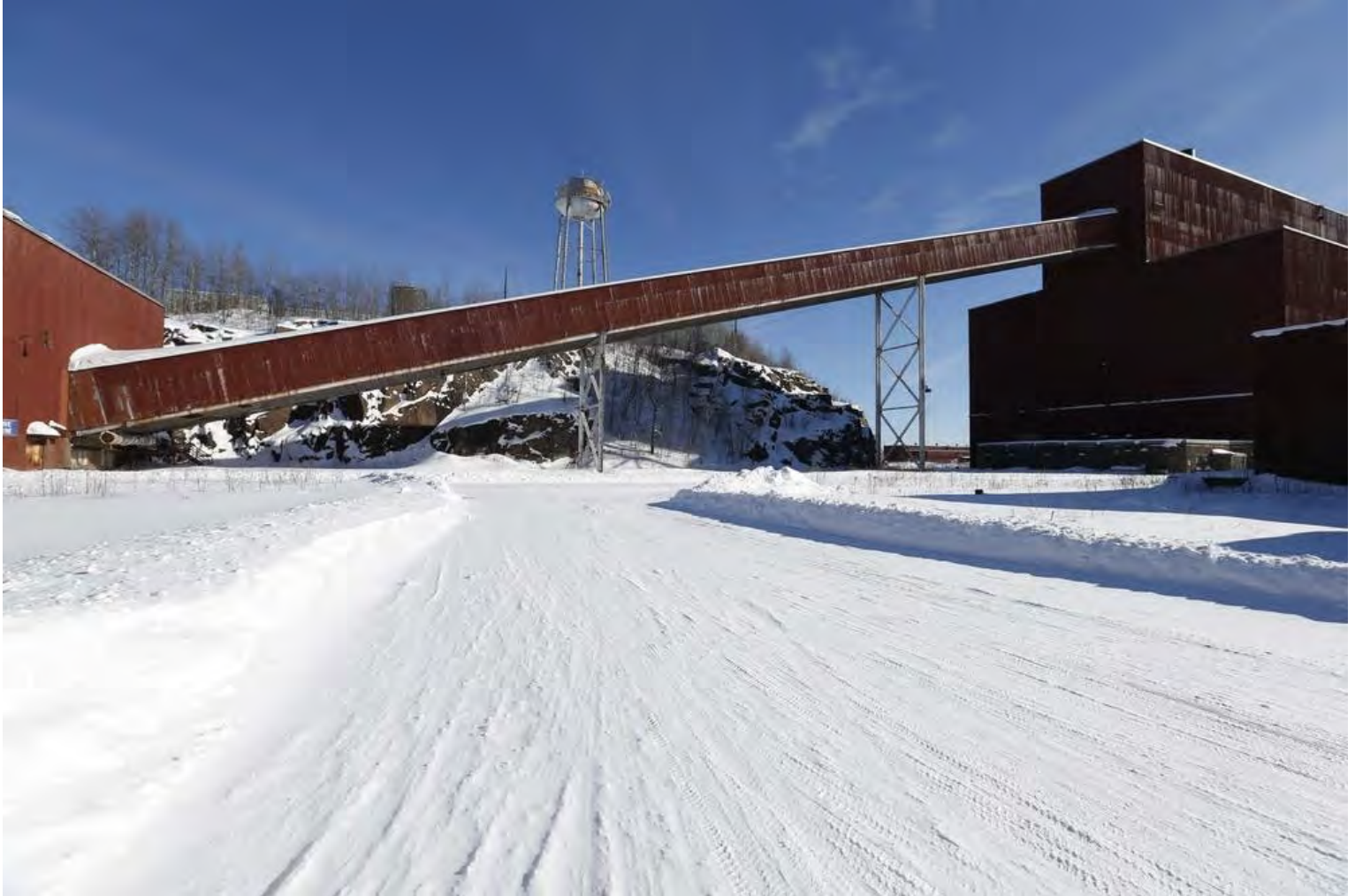
In this photo taken Feb. 10, 2016, the closed LTV Steel taconite plant is abandoned near Hoyt Lakes, Minn. Jim Mone | AP 2016
