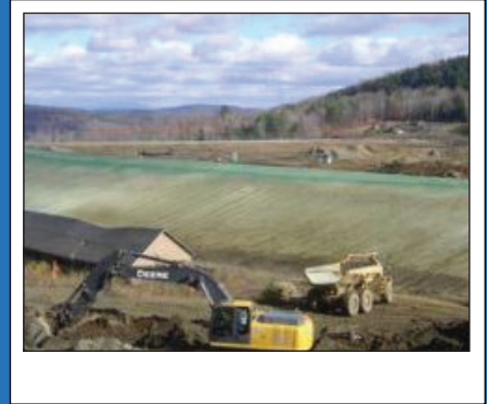
Elizabeth Mine stream and river restoration.
