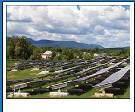
Stafford Hill Solar Farm.
