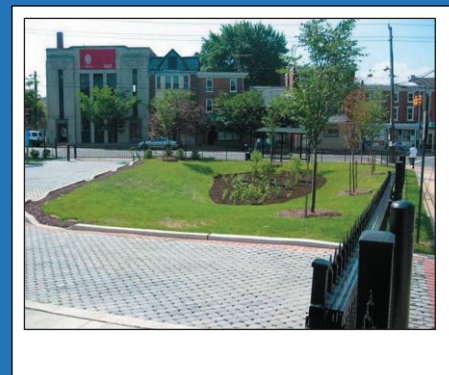
Bioswale and parking lot of the Brandywine Village Green.
