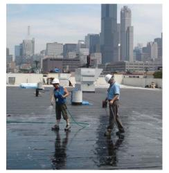
Image 20.1 Waterproofing membrane. Photo courtesy American Hydrotech, Inc.
