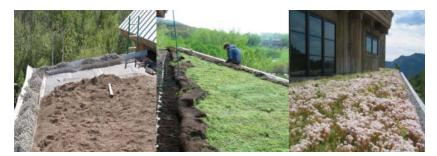
Photo 27.1 Example of 12" vegetation free zone at the perimeter of a green roof with vegetation mat. Photo on the right is one month after installation. Photo courtesy Andy Creath
