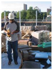
Image 15.1, Example of temporary dead and live loads during installation at the Gathering Place, Denver. Photo by Leila Tolderlund
