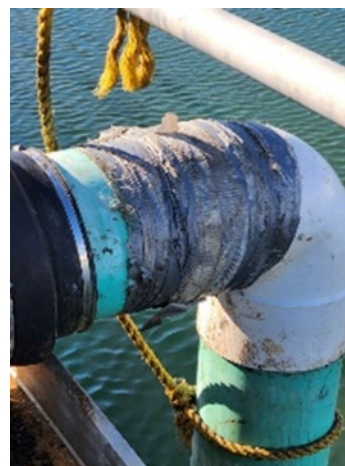
Example of poor maintenance of pipes using duct tape at the traditional side of the O.B. Curtis plant. (EPA OIG image).
