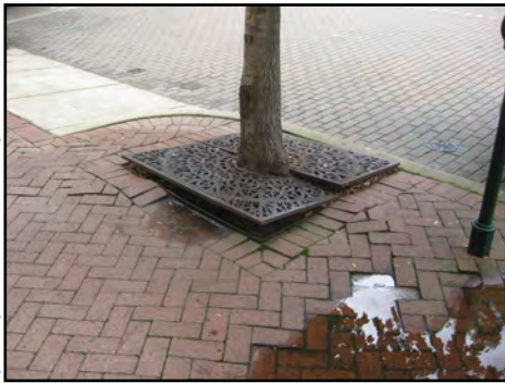
Figure 21. In many places, tree roots have grown beyond the tree wells, lifting pavers and creating tripping hazards for pedestrians.
