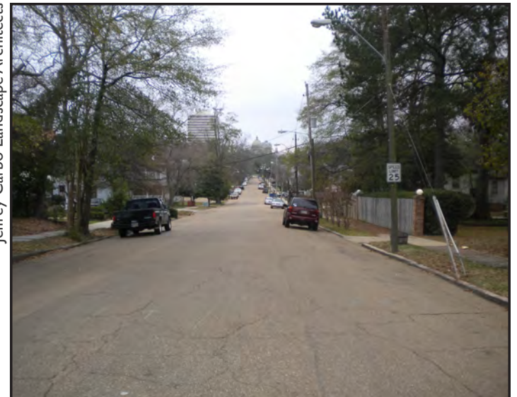
Figure 4. Existing conditions on North Congress Street.
