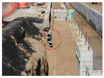
Figure 55: Construction photo showing utility conduits.
