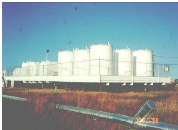
Figure 3-1: Fencing around oil storage area.
