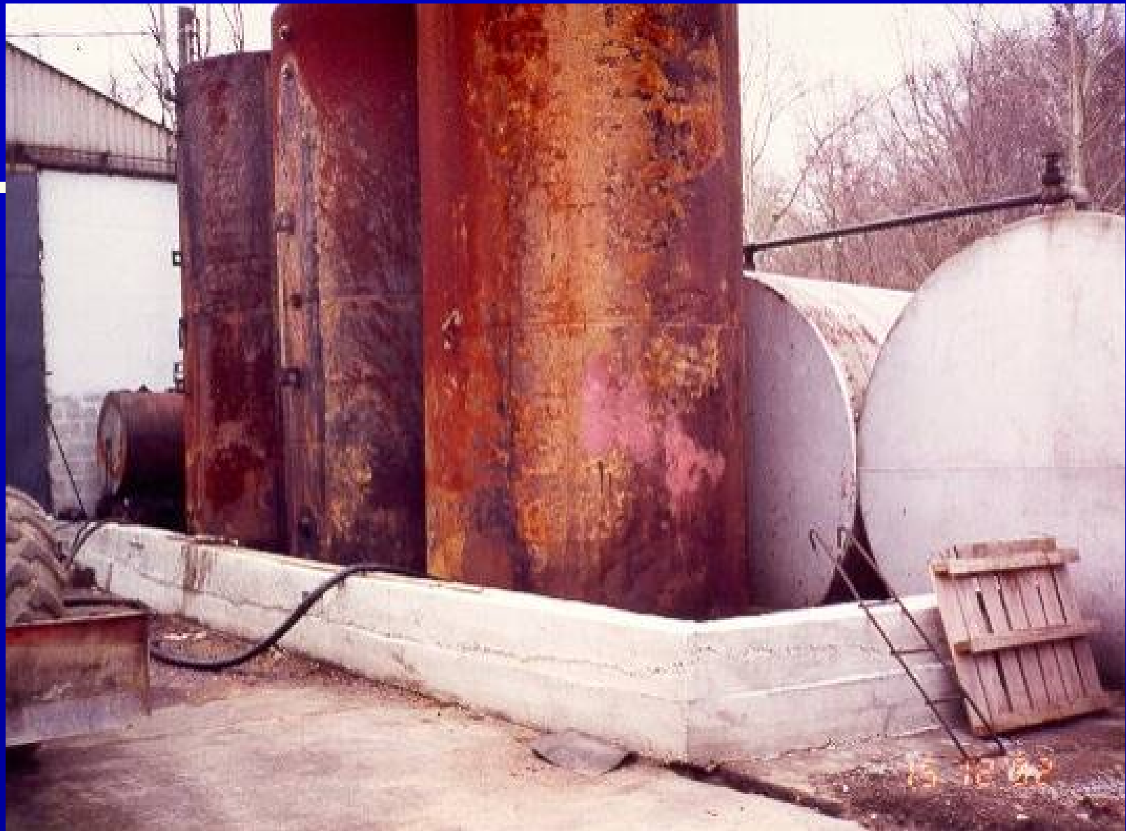
Inadequate Containment and Improper Tank Use (UST serving as an AST)
