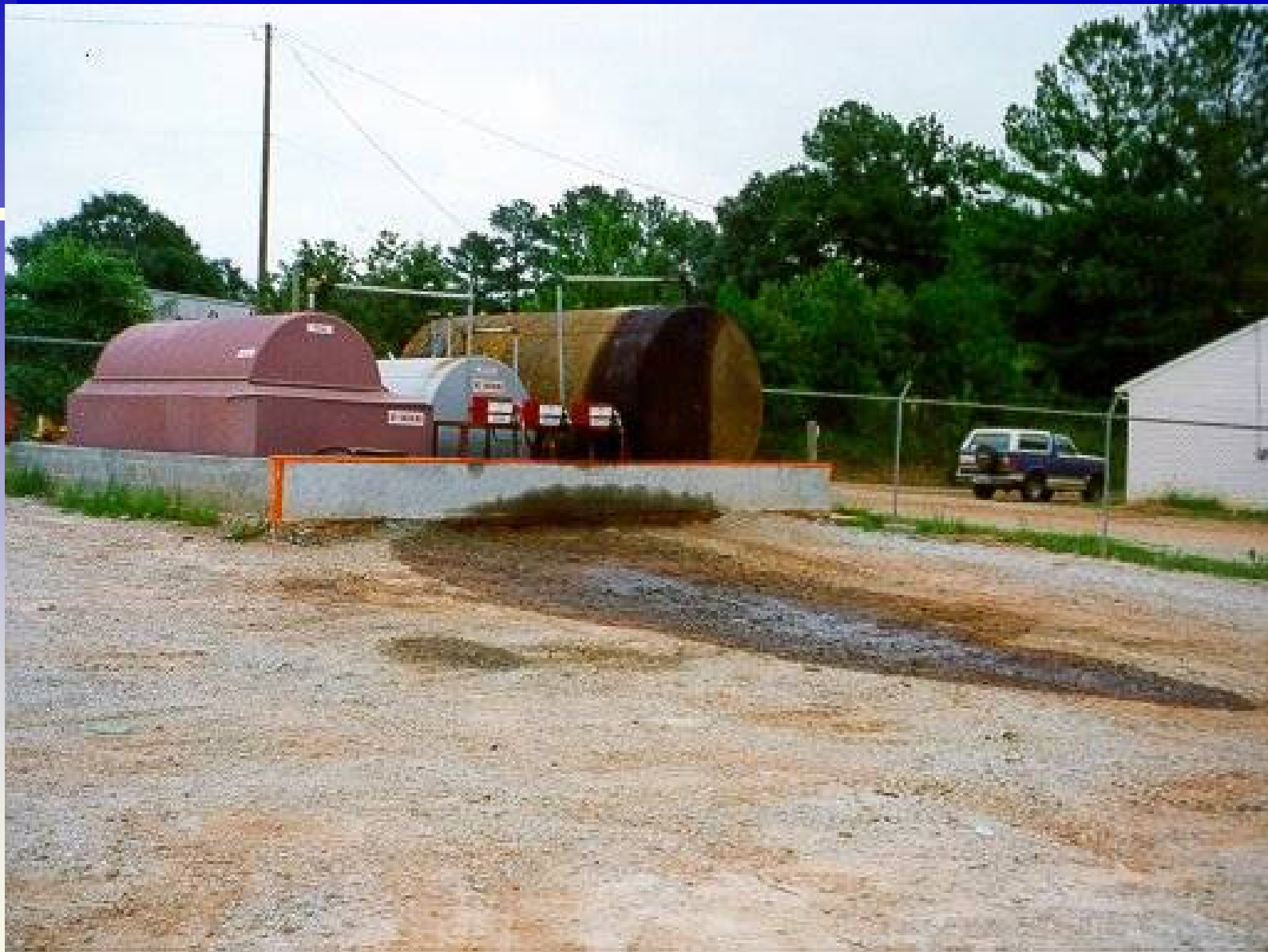
Inadequate Containment and Overfill Protection
