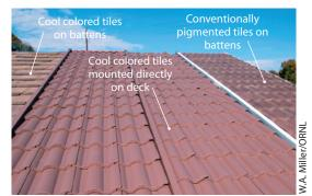
Cool roof products can be indistinguishable from their conventional counterparts. The rightmost row of curved tiles uses conventional colored pigments, whereas the other two rows use cool pigments. most common roofing materials used on steep-sloped roofs. Other products include metal roofing, tiles, and shakes.
