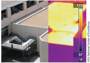
The left half of this traditional bitumen roof in Arizona is shown in visible wavelengths and the right in infrared. The roof's temperature reaches almost 175°F (80°C).
