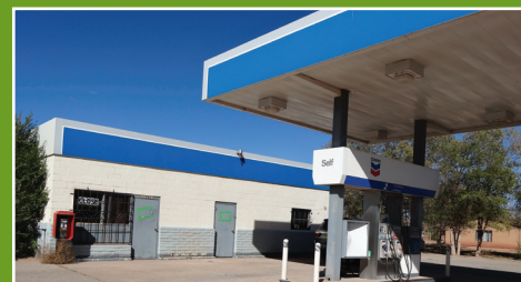
Closed Chevron gas station, Zuni Pueblo, New Mexico
