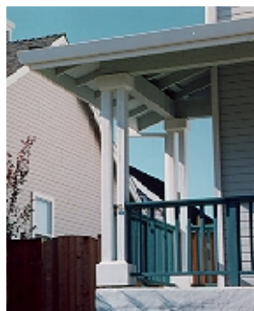
WELL PROPORTIONED AND DETAILED ENTRY COLUMN
