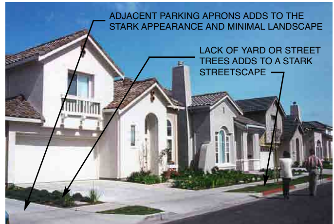
Undesirable: The lack of landscaping and large street or yard trees and the density of small lot developments has created a harsh streetscape in many recent projects.
