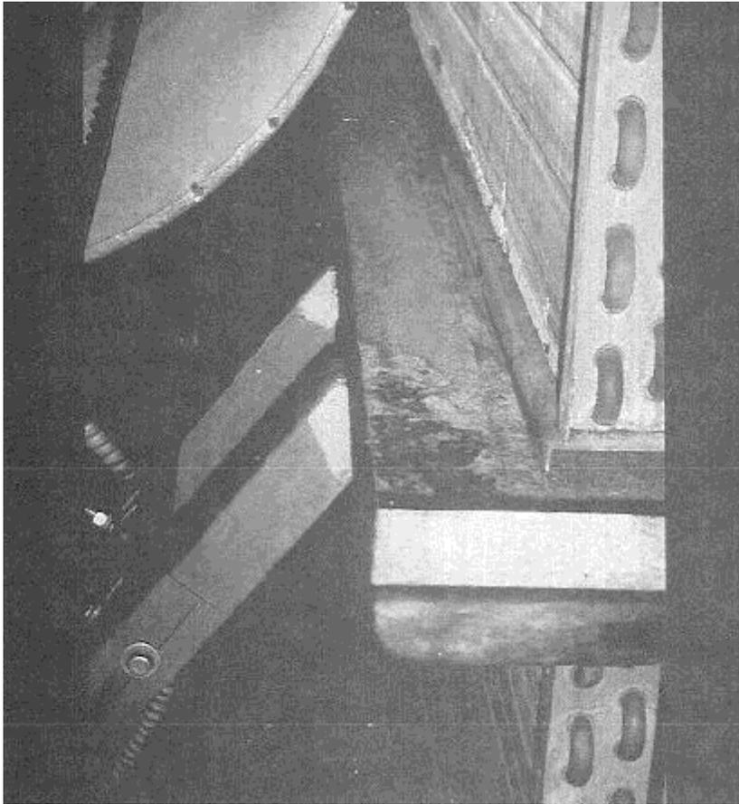
*Without proper installation and maintenance, rust and corrosion may accumulate in condensate pans under heating and cooling coils. The rust in the pan indicates that it was installed without a pitch or was pitched in the wrong direction, so that water did not drain out properly.*
