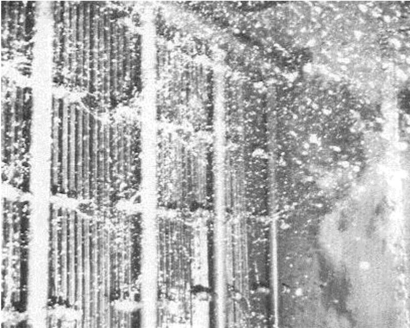
*This air washer is used to remove particles and water-soluble gaseous contaminants and may also control temperature and humidity in the airstream. Such systems are subject to severe bacterial contamination.*
