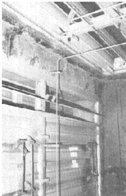
**Above:** The air intake in the background is located too close to the sanitary vents (the straight pipes to the left and in the center foreground) and the bathroom exhaust vent (next to the sanitary vent on the right side). **Below:** The return air dampers in this mixed-air plenum are open (top), but the outdoor air damper (left) is almost completely closed. Complaints in the building indicate that under-ventilation is a problem.
