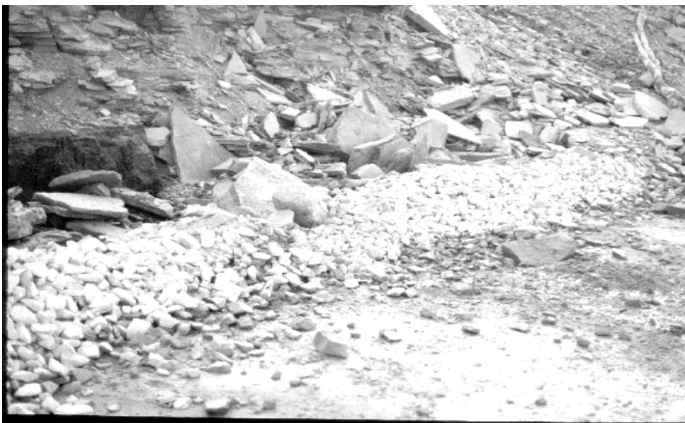
Figure 1.2.1i: Example of a Pit Floor Drain
