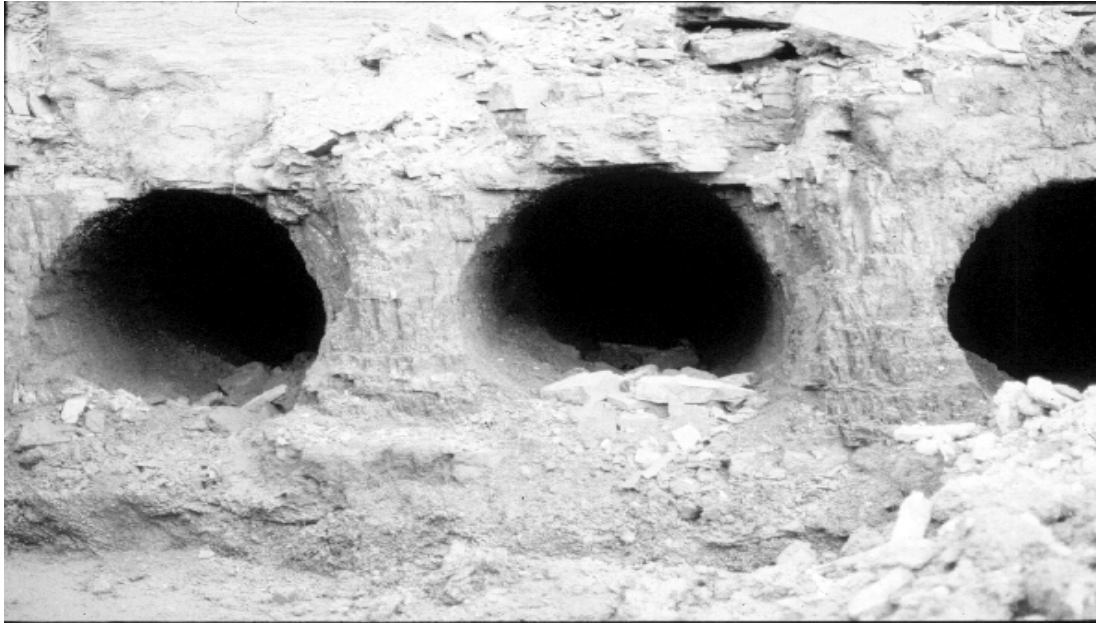
Figure 1.2.1b: Exposed Auger Holes
