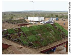
This home in Arizona shows a modular green roof on a steep-sloped roof.
