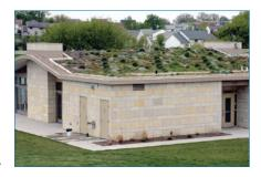
Both cool and green roofs lower surface and air temperatures and reduce summertime peak and overall energy demand. The extent of the energy savings varies depending on factors including the local climate, attic ventilation and insulation levels,
