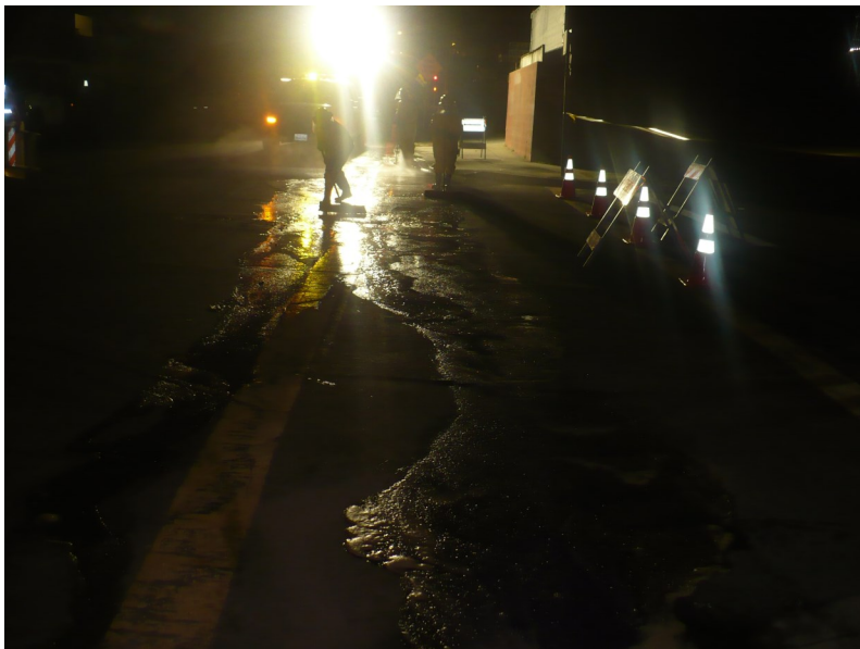
The cleanup of the acid spill outside Pacific Tank Cleaning, Inc.
