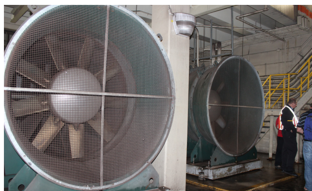
NYC Subway Ventilation Fans
