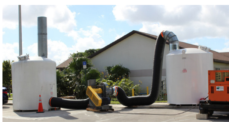
Activated Carbon Scrubber
