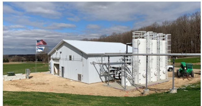
Biogas upgrade equipment at Clover Hill Dairy. Photo Credit: DMT Clear Gas Solutions
