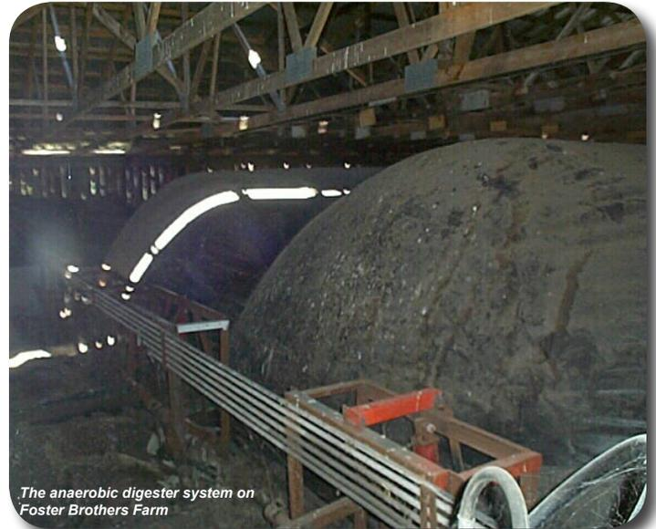
The anaerobic digester system on Foster Brothers Farm
