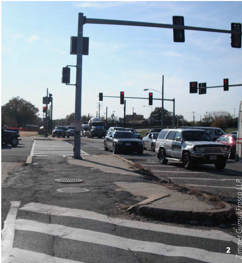
Figure 18: Though each of the free right turn lanes on Suitland Parkway has a small refuge, they are badly deteriorated and do not meet accessibility standards.
