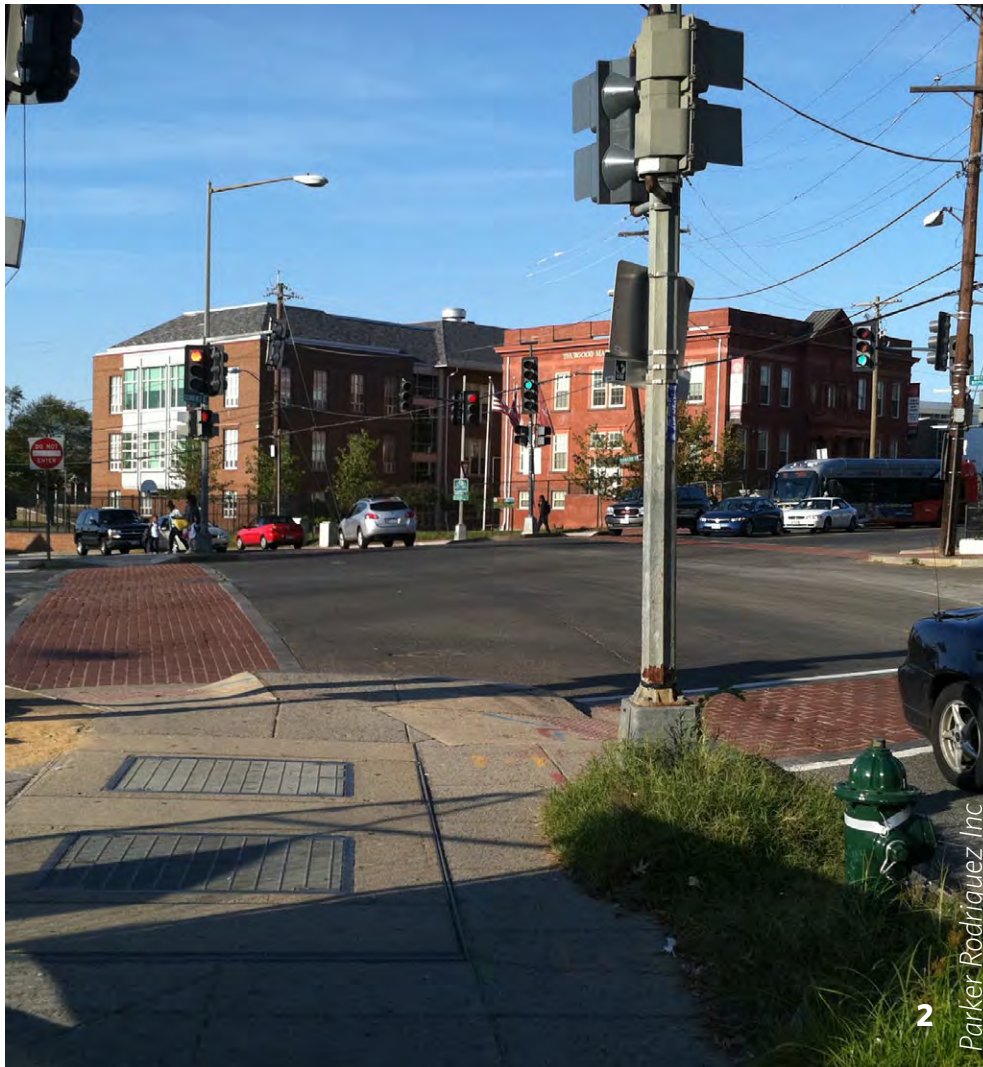
Figure 22: The five-way intersection of MLK Avenue, Howard Road, and Sheridan Road is confusing, and crossing distances are long due to angled crosswalks.
