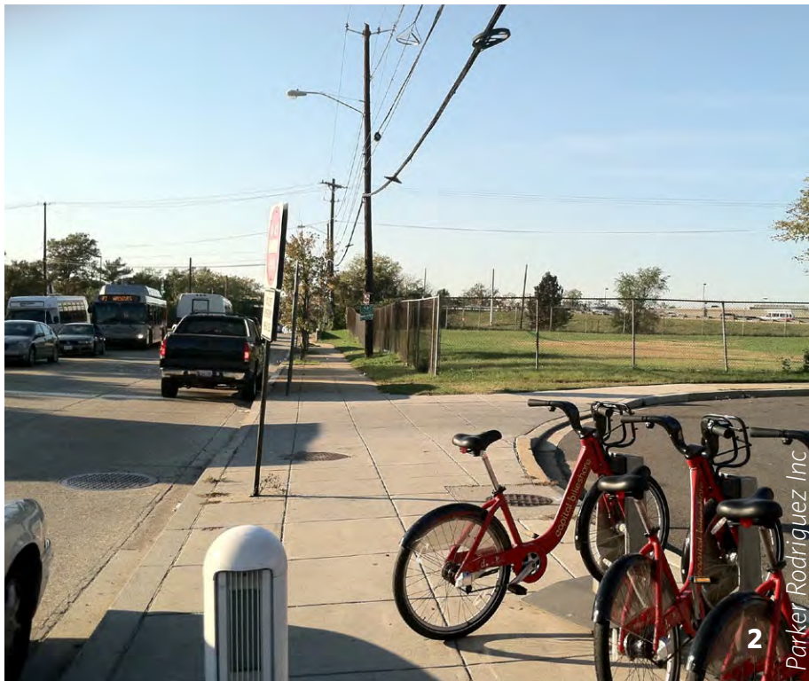
Figure 14: A rolled curb on Howard Road at Shannon Place allows emergency access, but many motorists drive over the sidewalk, endangering pedestrians.
