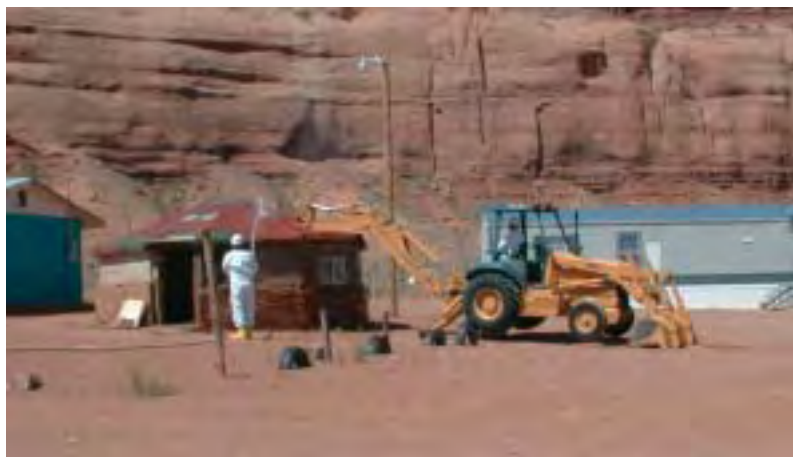
Above: EPA and the Navajo Tribe demolished and removed this traditional dwelling on the Navajo Nation because it was made of radioactive rock and soil from a uranium mining area. It was being used for storage. Photo by Andrew G. Sowder. Below: Supply Creek Open Dump before closure, on Hoopa Valley tribal land, Northern California. Photo courtesy of Hoopa Valley Tribe.
