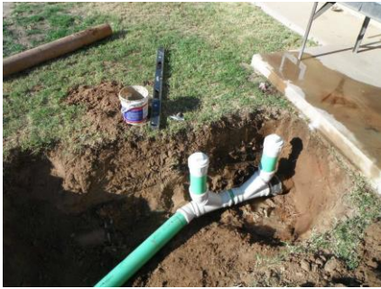
Work at the Holtville wastewater collection project
