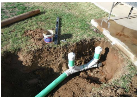
Work at the Holtville wastewater collection project
