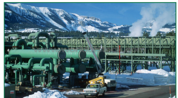
A geothermal power plant in Mammoth Lakes, CA
