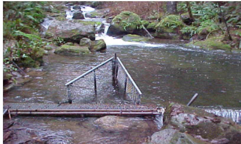
A Drinking Water Intake for a Surface Water System
