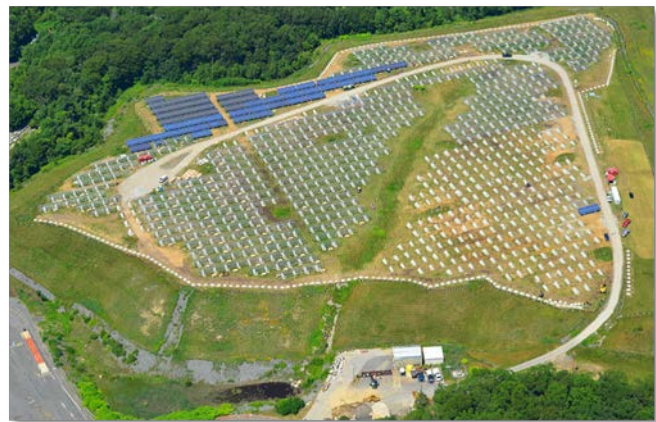
Scituate Landfill solar under construction. Courtesy Brightfields Development LLC
