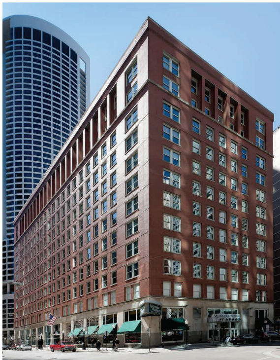
The Railroad Retirement Board is in the Lipinski Federal Building in Chicago.
