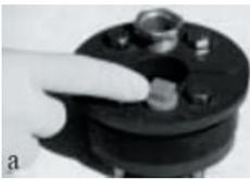
Determine what type of well you have and how to pour the bleach into the well. Some wells have a sanitary seal with either an air vent or a plug that can be removed (a). If it is a bored or dug well, the entire cover can be lifted off to provide a space for pouring the bleach into the well (b).
