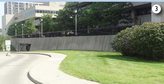
Figure 18: Retaining Wall Looking Northeast
