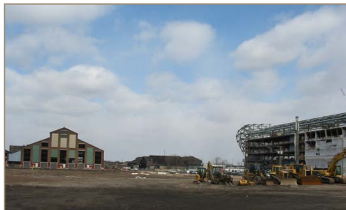
Hudson County Assessment grant's new stadium under construction in New Jersey
