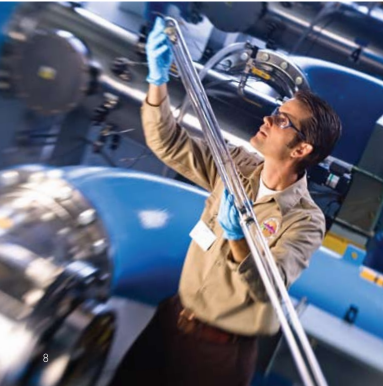
Bryan (Water Facilities Operator, Department of Utility Services) maintains the ultraviolet light chambers that assist in disinfecting our water supply.
