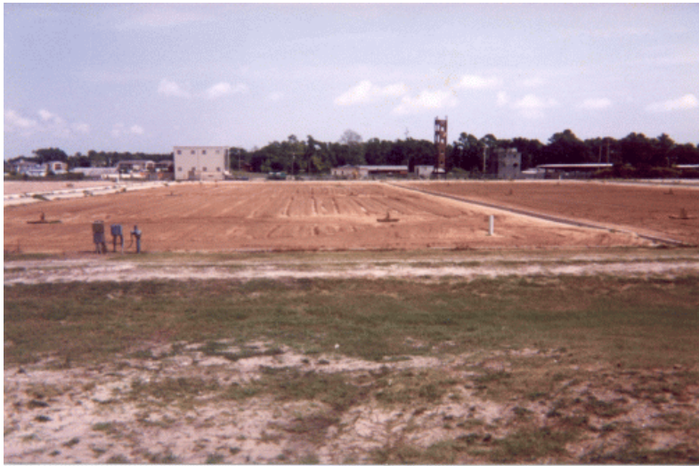
Intermittent Sand Filters
