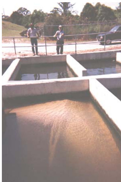
Sand Accumulation in Chlorine Contact Chamber
