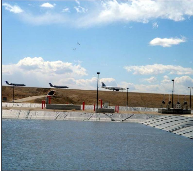
**Figure 7-3. Pond for Deicing Stormwater Storage**
