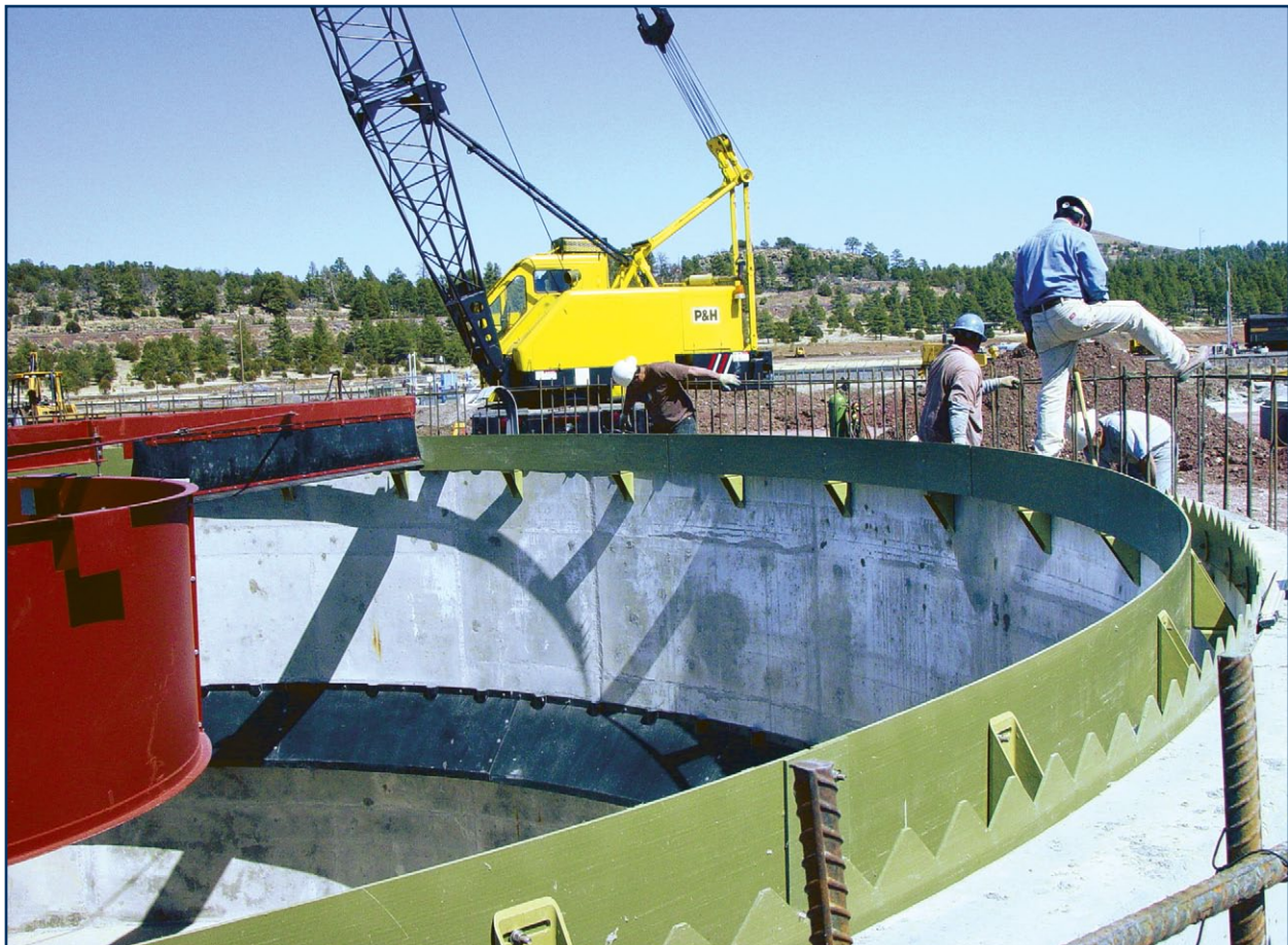
City of Williams, Arizona. Construction of Clarifier. Courtesy of Water Infrastructure Finance Authority (WIFA) of Arizona.
