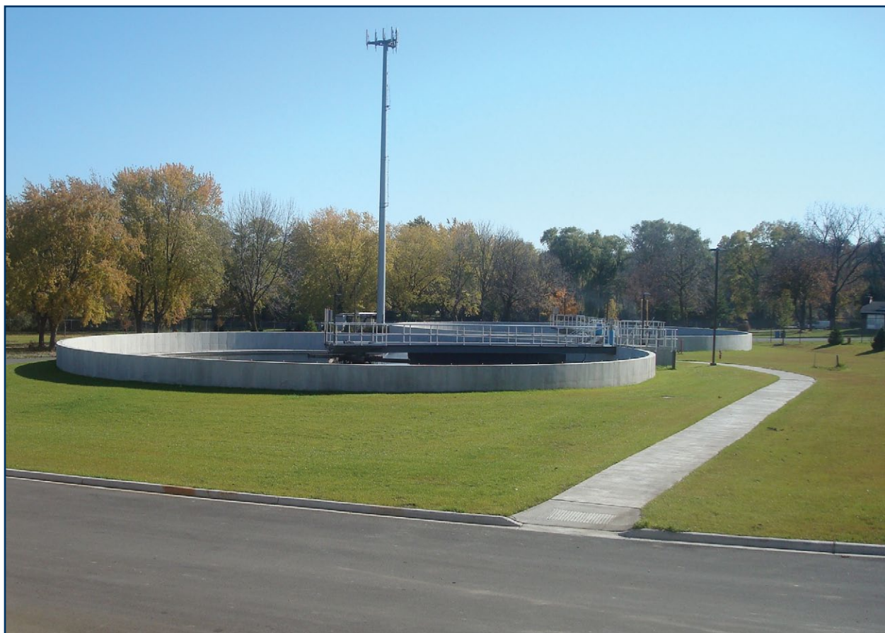
Village of Algonquin, Illinois. Aeration basin and secondary clarifier. Courtesy of EPA Region 5.
