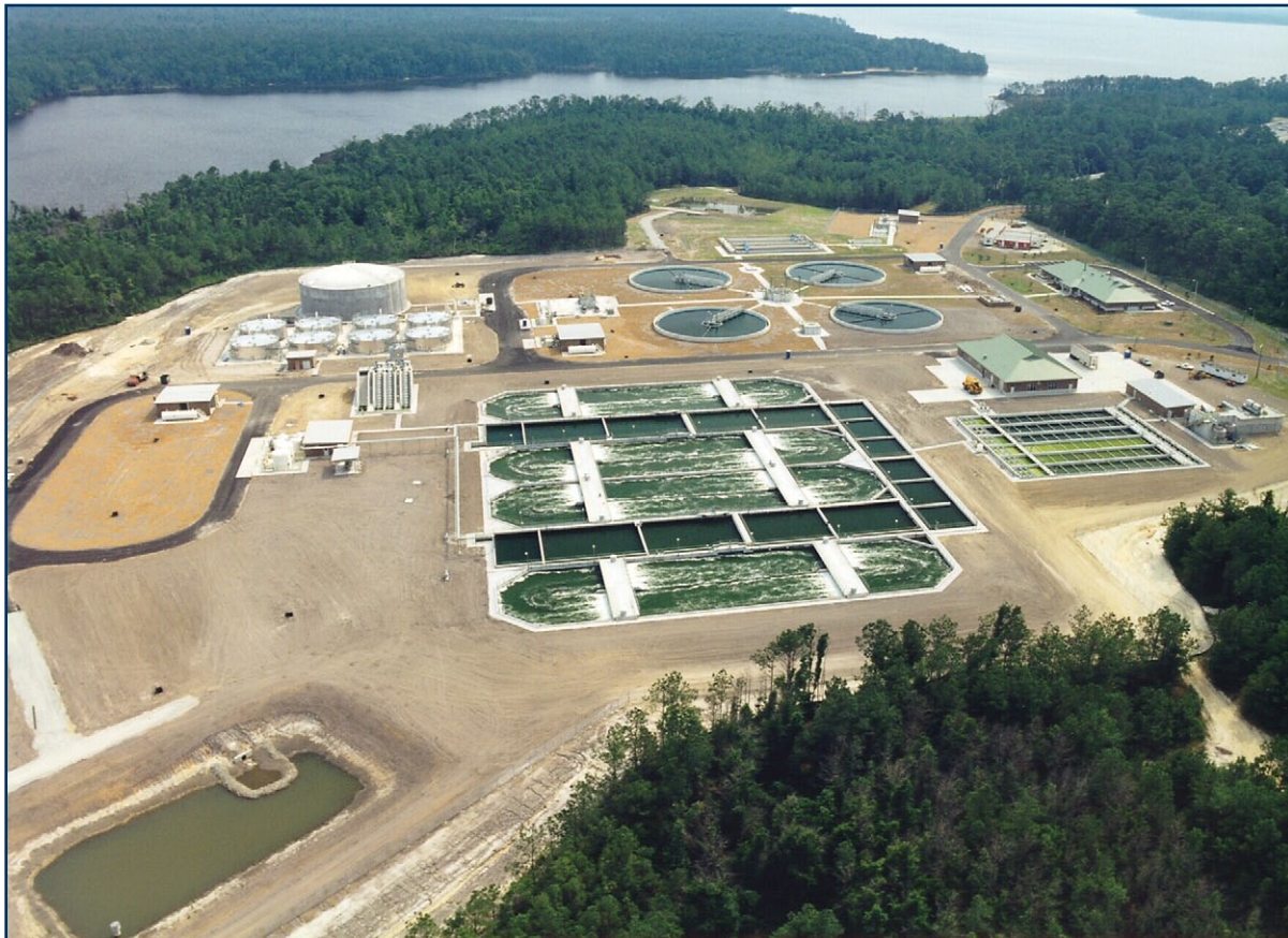
Wastewater Treatment Plant, Jacksonville, North Carolina.
