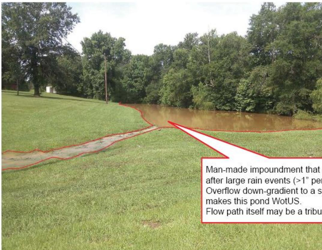
Man-made impoundment that overflows after large rain events (>1" per hour). Overflow down-gradient to a stream makes this pond WotUS. Flow path itself may be a tributary
