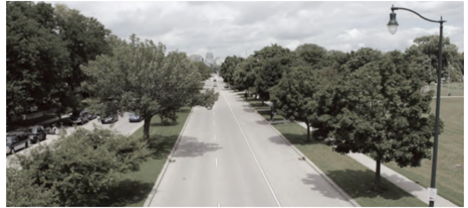
FIGURE 18 Existing view looking northeast along West Washington Avenue toward the capitol building. As noted at the workshop, crossing West Washington Avenue at grade is unsafe, and the street currently has no identified pedestrian crossing.
