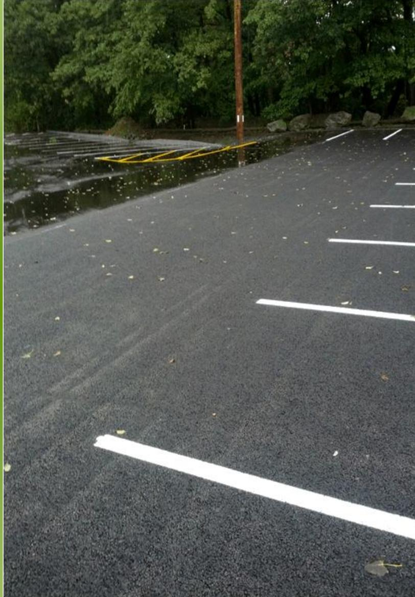
Photo taken during rainstorm showing comparative performance of traditional pavement (left) and porous pavement (right)
