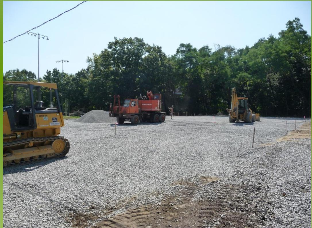
$\frac{3}{4}$ " Crushed Stone Grading
