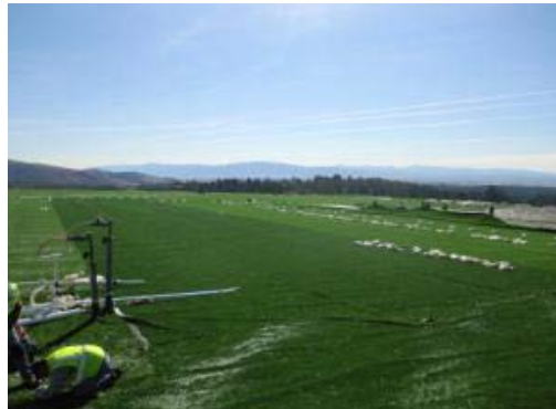
Crazy Horse Landfill Deemed Suitable for Solar Photo credit: Blaise Stoltenberg, NREL
