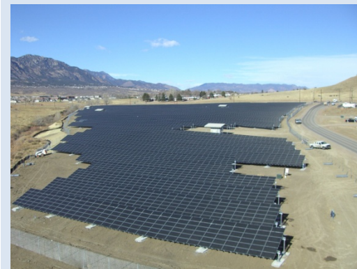
An Example of a Solar Photovoltaic Facility on a Former Landfill in Fort Carson, Colorado
